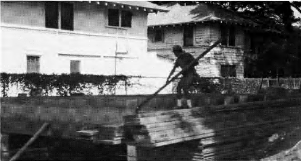
The foundation being built. The old residence in the background, right.
