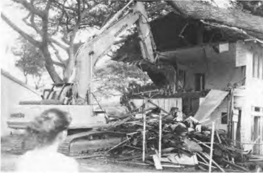
Ashley Dutro watches as her old home is demolished.
