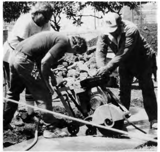
Peter Pasigan, Harry Marchadie and Tovia Fatu working concrete saw.
