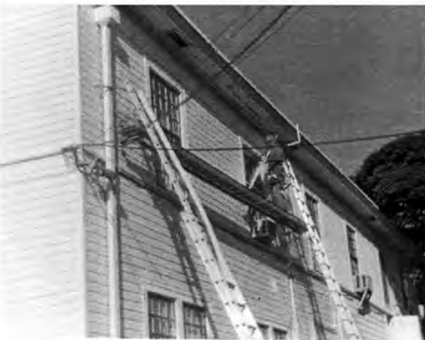
Vinyl siding being put on the Tenant Building.
